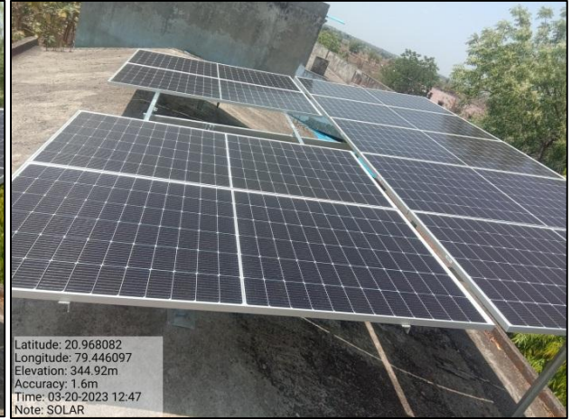
Solar Panel installed at the roof top of college building
