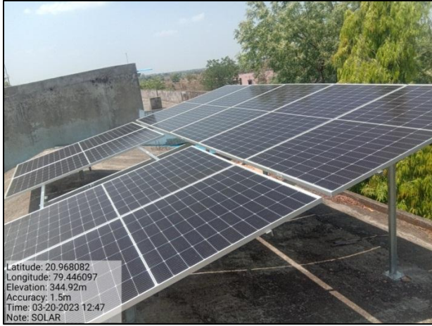
Solar Panel installed at the roof top of college building
