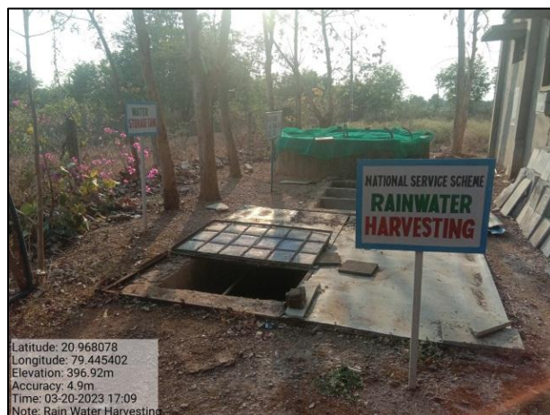
Systematic arrangement of rainwater filtration with recharge facility
