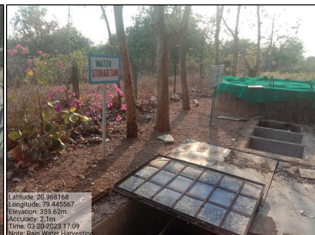
Systematic arrangement of rainwater filtration with recharge facility
