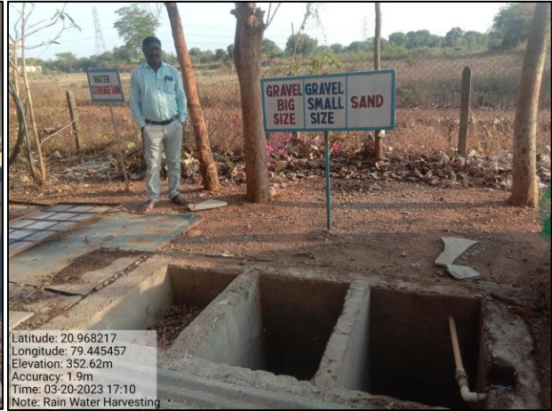
Filtered rainwater connected to collection area
