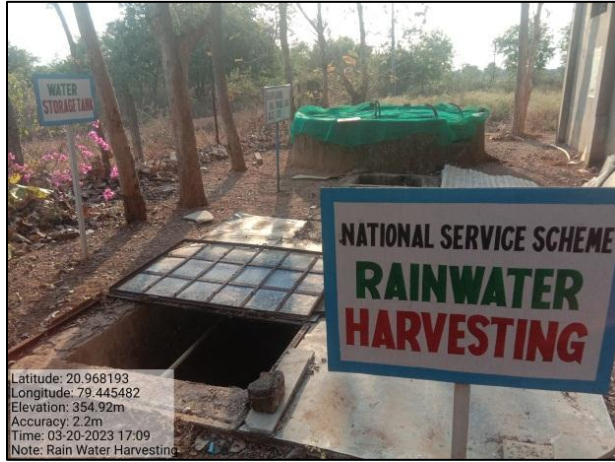
Filtered rainwater connected to collection area
